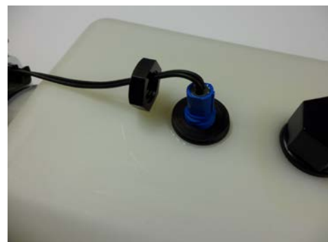
Figure 10 Float switch installation
