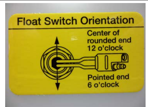
Figure 11 Label on side of vertical tank
