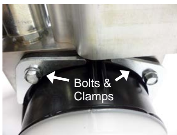
Figure 15 Bolts and clamps (4) on tank flange
